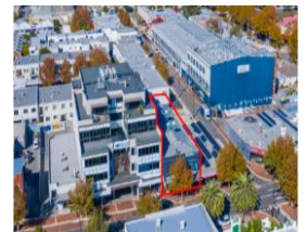
Existing Asset Refurbishment Western Australia 1 st Mortgage $2.0m
