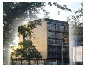
Existing Asset Refurbishment Victoria 1 st Mortgage $6.2m
