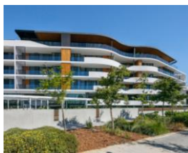
Post-Construction Residual Stock Western Australia 1 st Mortgage $16.8m
