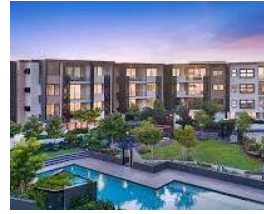
During Construction Development Queensland 2 nd Mortgage $2.8m
