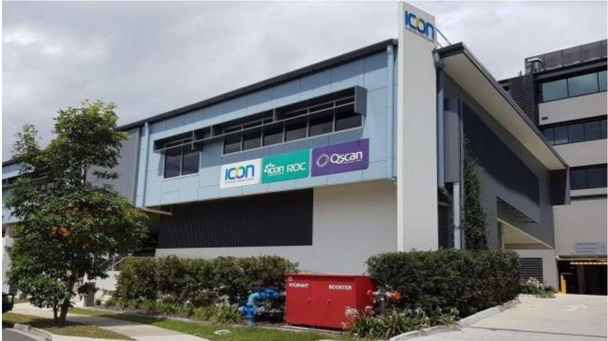
The North Lakes medical facility in Queensland which Barwon has acquired for its institutional healthcare property fund.
