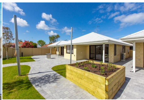
South Bunbury SDA House / Villas, WA
